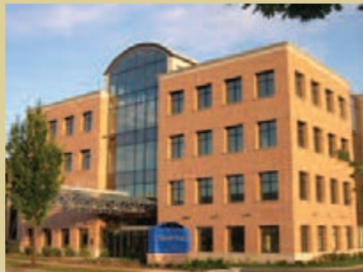
Summit Place office complex PHOTOS COURTESY CITY OF WEST ALLIS
