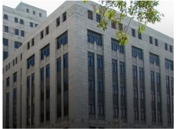
The State Human Services Building at 1 W. Wilson St. now faces more than $228 million in projected upgrade and renovation costs.
