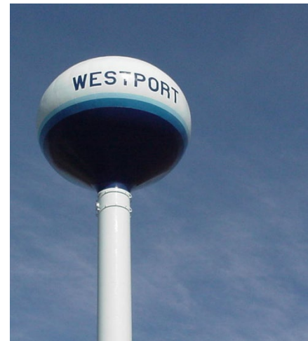
Figure 63: Mary Lake water tower, Town of Westport.
