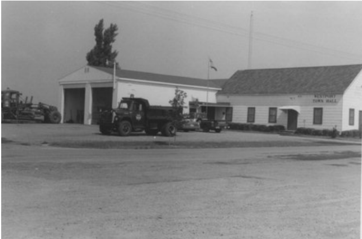
Figure 15: In July 1977 the Westport Town Hall was in a smaller building located where the parking lot and driveway currently exist just south of the current public works garage. These structures were demolished in 2014. Source: Wisconsin State Historical Society.
