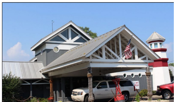
Figure 44: The former Mariner's Inn Restaurant, demolished in 2026, originally opened in 1966. Source: Waunakee Tribune, August 13, 2025; photo credit: Roberta Baumann.
