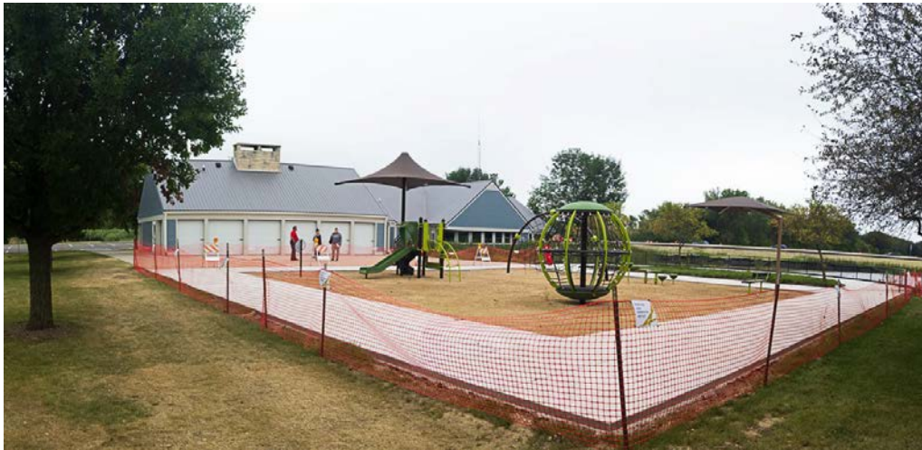
Figure75: Westport Town Hall and Town Center Park Playground under construction.
