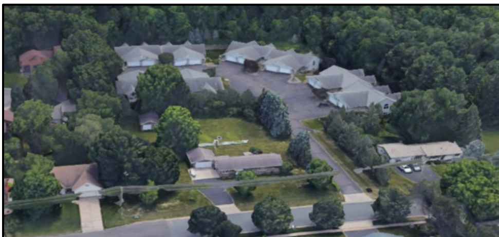
Figure 30: Foxwood Condominiums on McElroy Court
