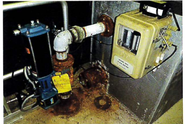
Figure 6.01-11 DAFT Flow Measuring
