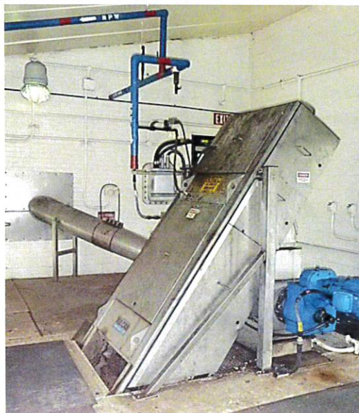
Figure 6.01-3 Mechanical Step Screen
