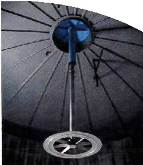
Figure 7.02-7 Example LM Mixer Installations
