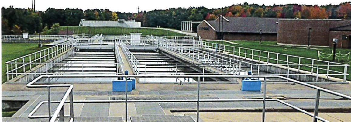
Figure 6.01-6 Primary Sedimentation Tanks
