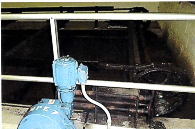
Figure 6.01-10 DAFT Chains and Sprocket
