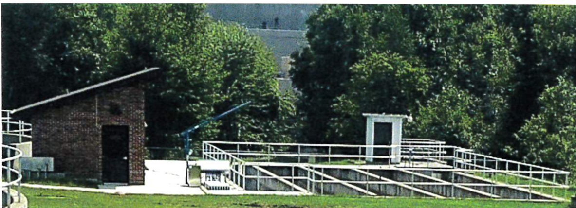
Figure 6.01-9 UV Disinfection and Postdisinfection Settling
