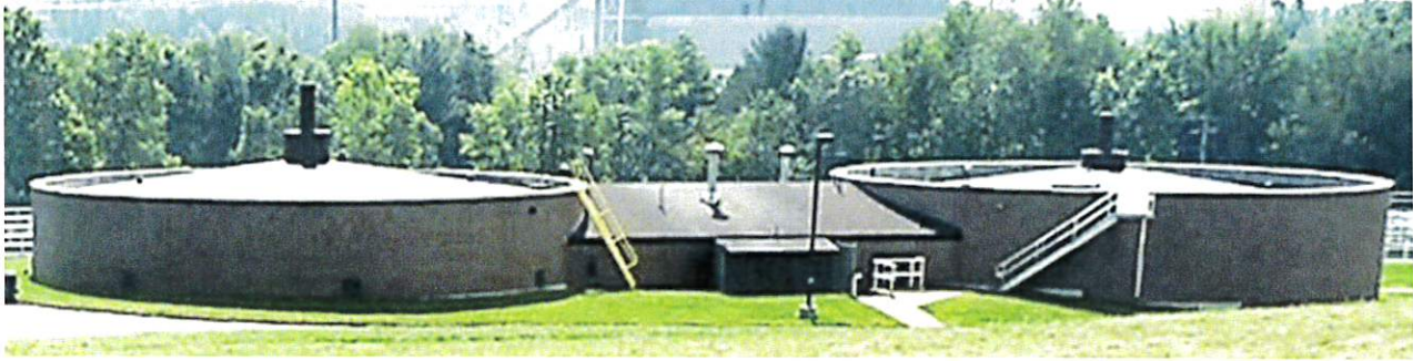
Figure 6.01-12 Anaerobic Digesters
