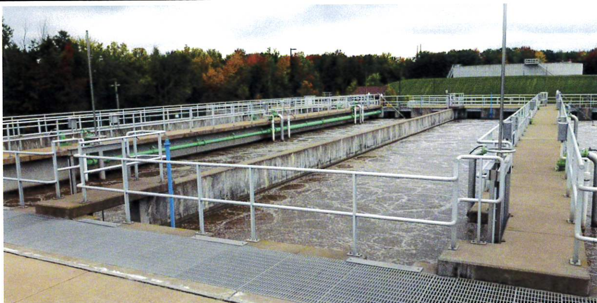
Figure 6.01-7 Aeration Tanks
