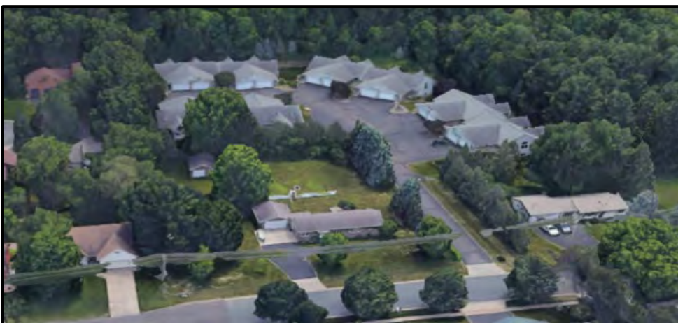
Figure 30: Foxwood Condominiums on McElroy Court
