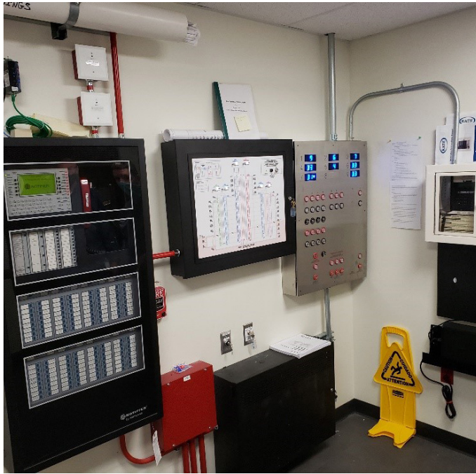
Fire Alarm Control Panel in Fire Command Center
