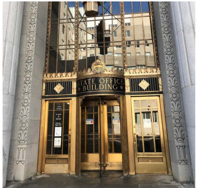
Existing bronze revolving door will need to be replaced
