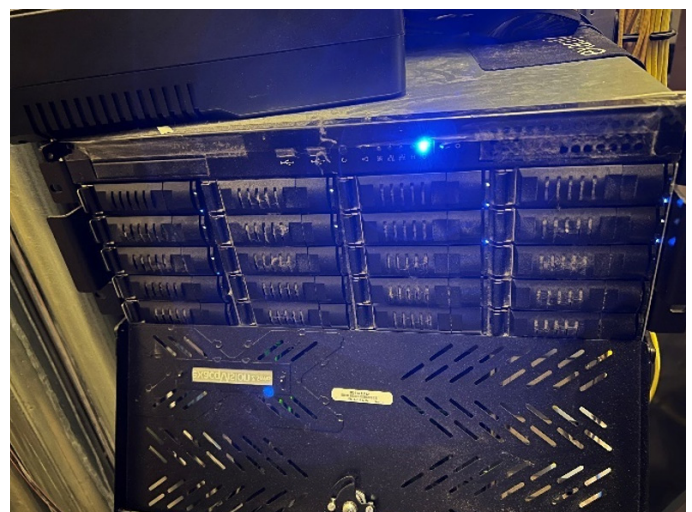
The existing Exacq Vision network video recorder located in Telecommunication Room 154Z
