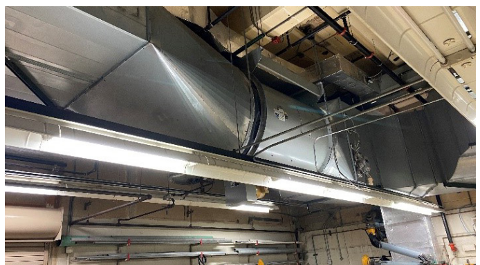
Typical inline exhaust fan
