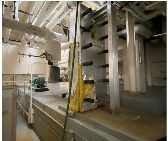
Existing heat recovery system heat exchanger abandoned in place
