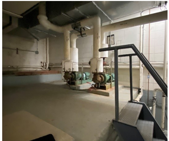
Existing heat recovery system pumps and piping abandoned in place
