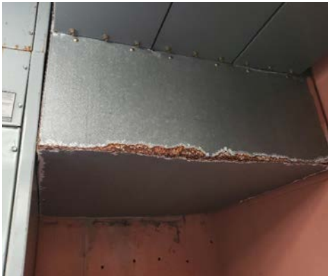
Moisture degradation of Electrical Service Equipment
