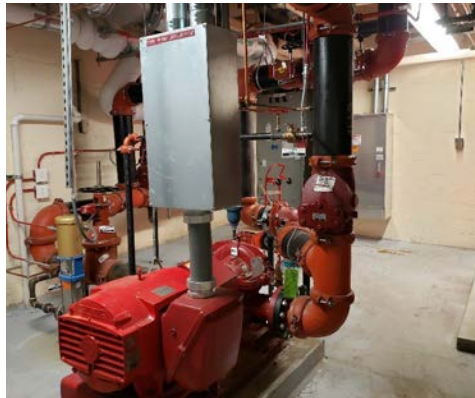
Fire Pump with service equipment
