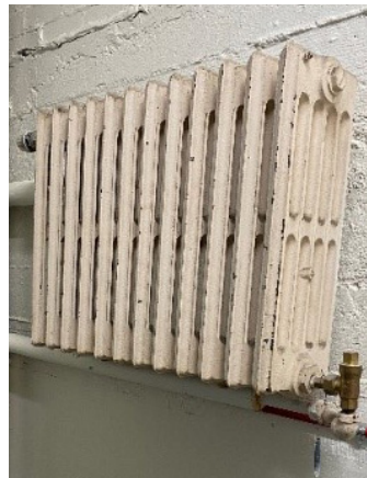
Typical steam original cast iron radiator; Typical radiator replaced with convector
