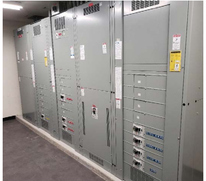
Generator Switchboard
