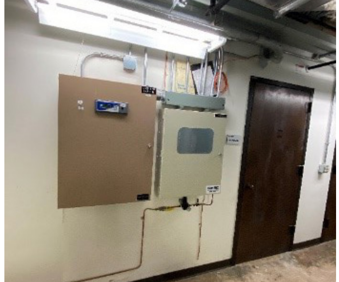
New DDC panel next to old pneumatic panel
