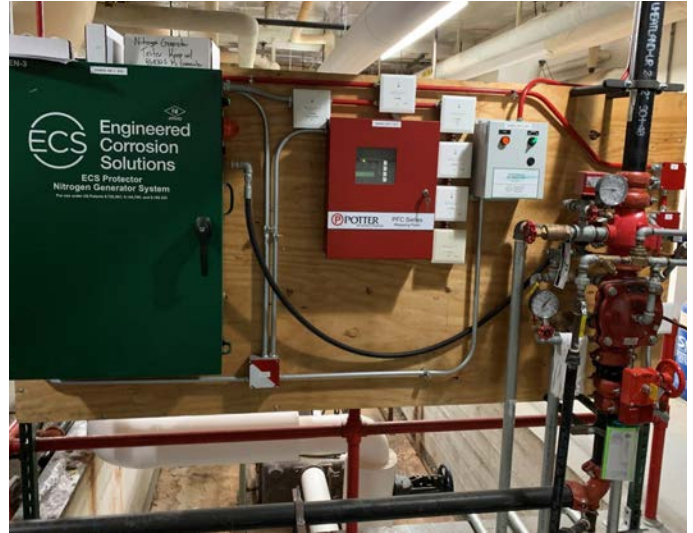
Double Interlock Preaction System with nitrogen on B3
