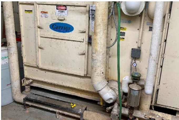
Example of old AHU with no access between heating and cooling coils or humidifier
