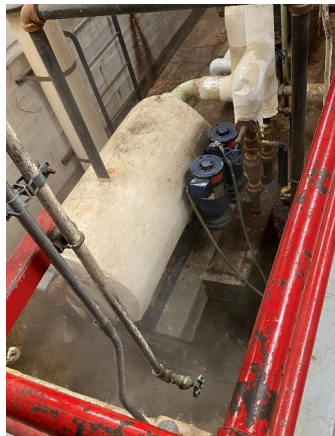
Typical condensate transfer pump in pit; Typical vacuum pump unit in pit
