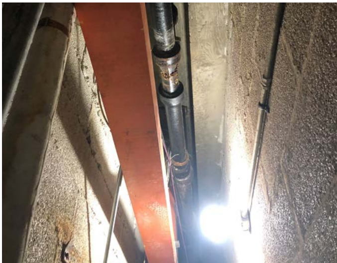
Condition of cast iron piping (note: this vertical plumbing chase will need to be infilled at each floor)
