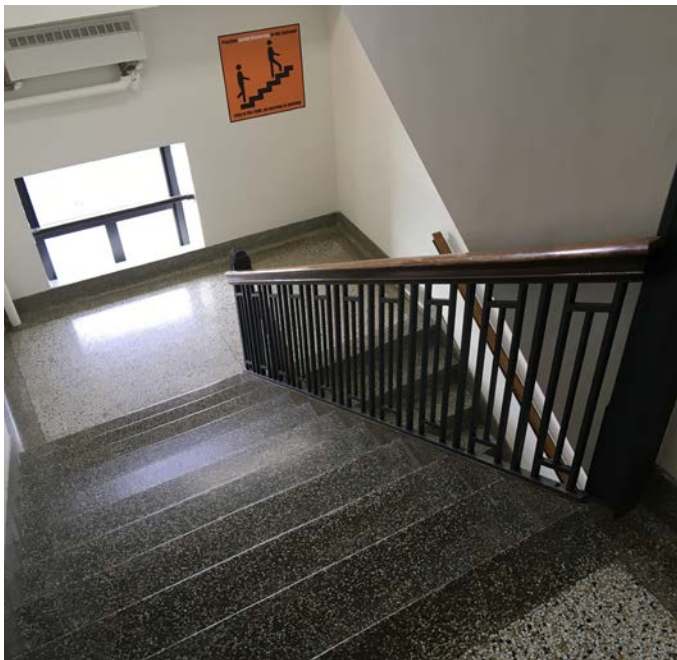
Existing Stair towers feature terrazzo and are in good condition
