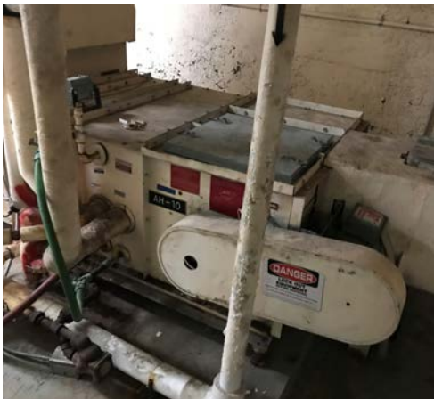
Example of decades old air handler that needs to be replaced
