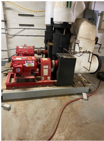
Building Chilled Water Pumps
