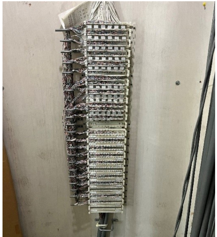
Category 3 Termination located in Telecommunication Room 272Z
