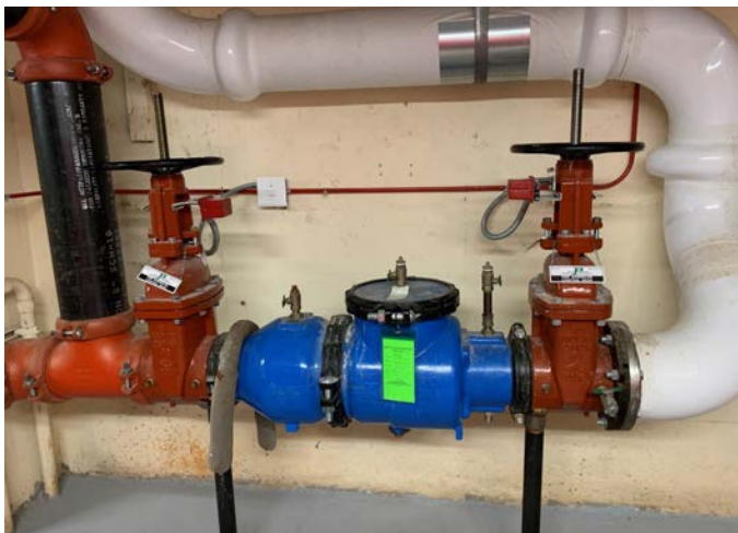
Double check backflow preventer in fire pump
