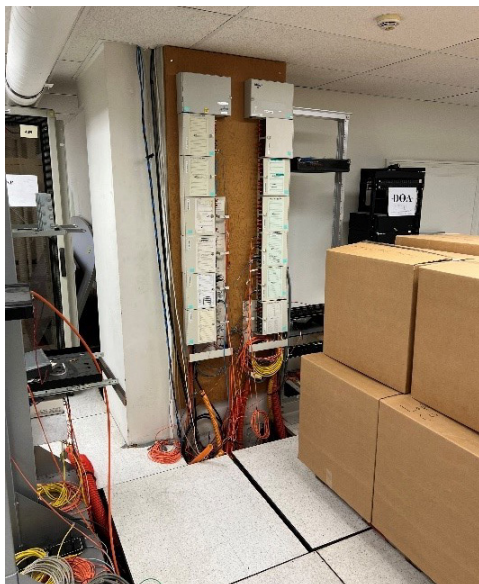
Inter-building Fiber Optic Cabling Terminations (Computer Room B218)
