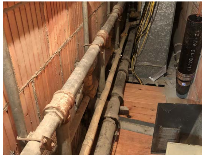
Condition of cast iron piping (note: this vertical plumbing chase will need to be infilled at each floor)
