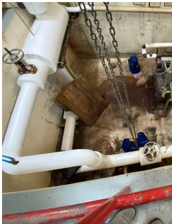
Typical condensate transfer pump in pit; Typical vacuum pump unit in pit
