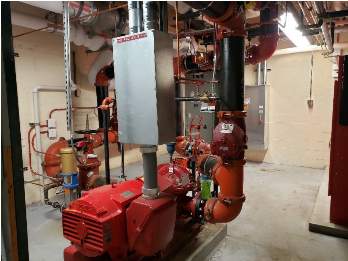
Fire Pump with service equipment
