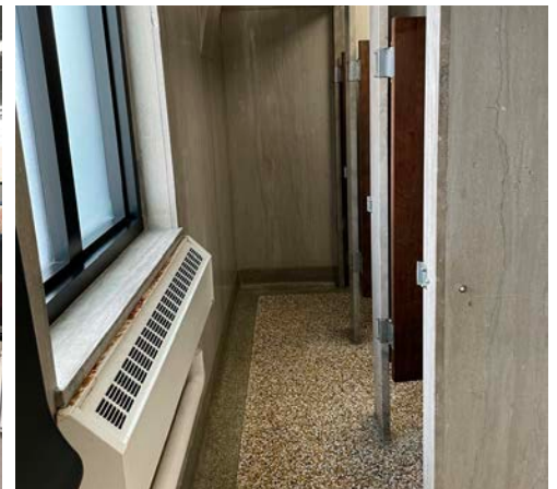
Example of existing inaccessible restroom
