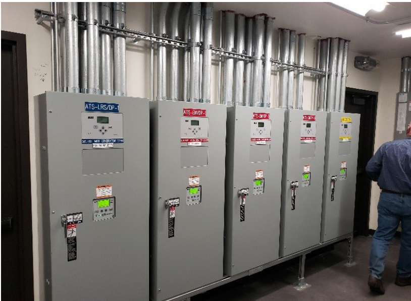
Automatic Transfer Switches
