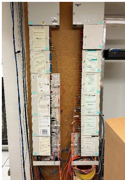
Inter-building Fiber Optic Cabling Terminations (Computer Room B218)
