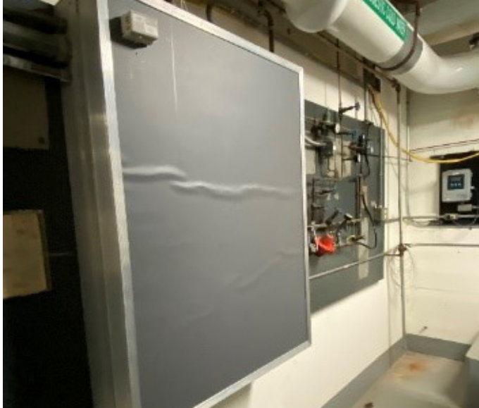
Original pneumatic control panel
