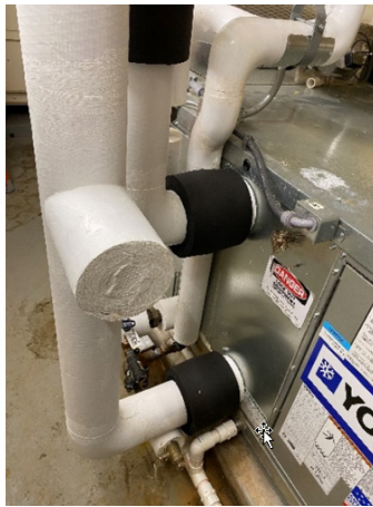
Newer Chilled Water Piping
