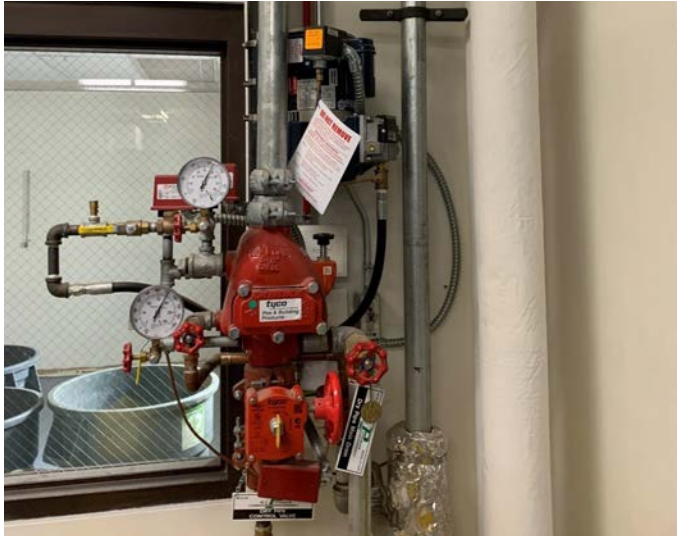
Dry-pipe valve at loading dock
