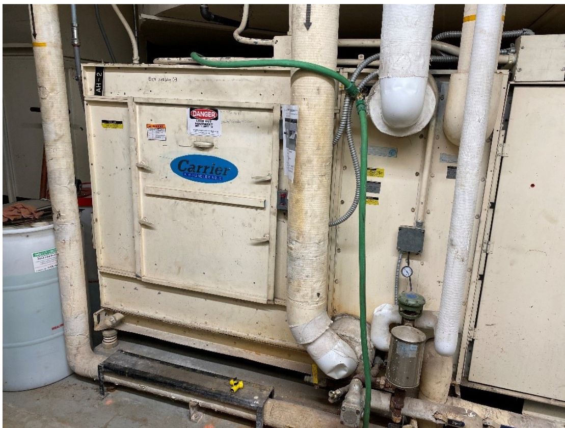
Example of old AHU with no access between heating and cooling coils or humidifier
