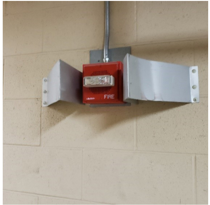
Audible Visual Fire Alarm Device
