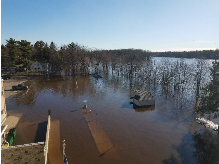
2019 Flooding at WRSOB
