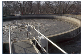
Waste Water Treatment Facilities/Plants (WWTF/P)
