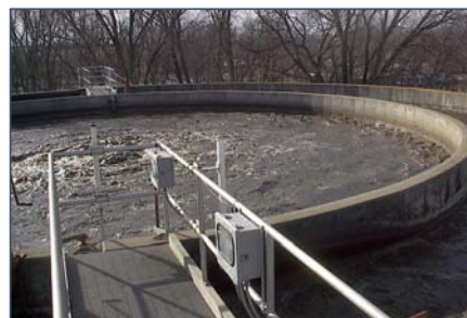
Waste Water Treatment Facilities/Plants (WWTF/P)
