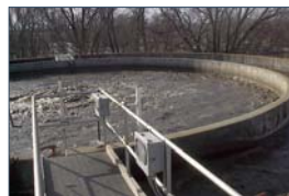
Waste Water Treatment Facilities/Plants (WWTF/P)
